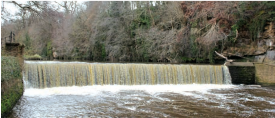
Dowie's Mill Weir
